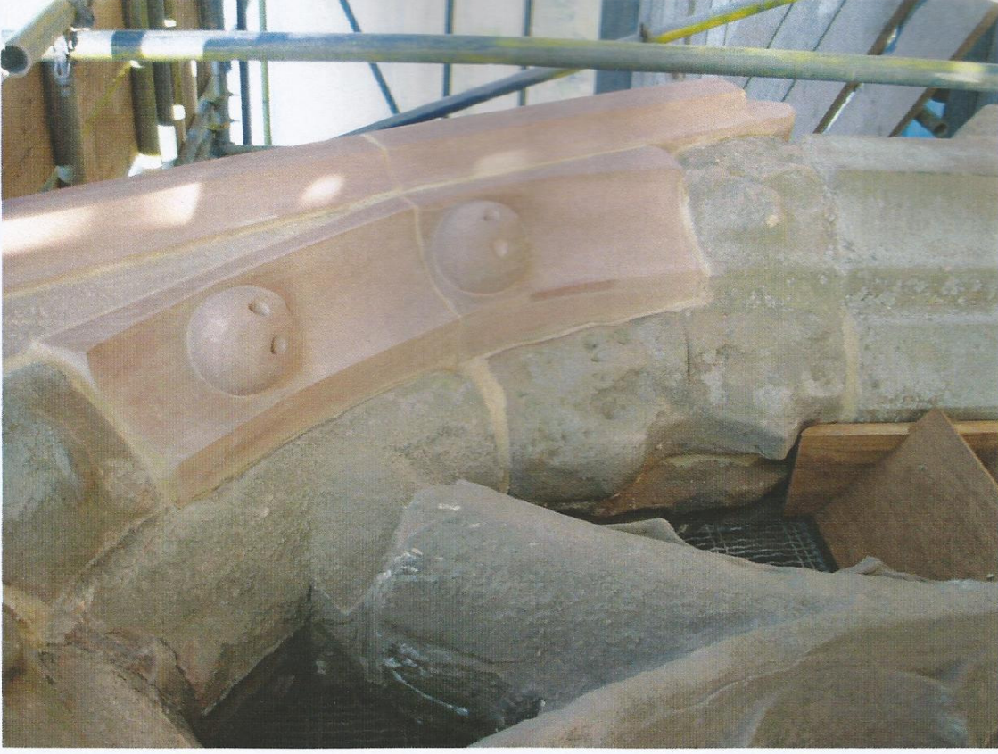
2. Renewed stonework to gablet of spire light
