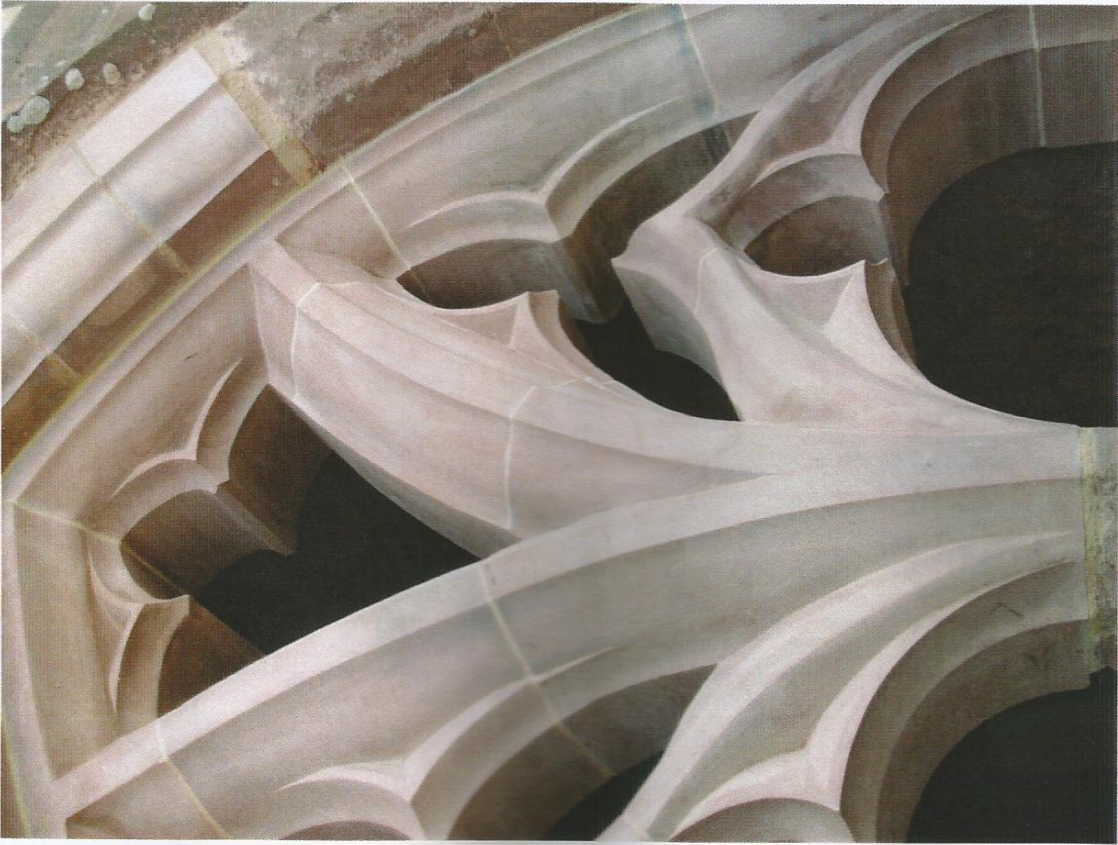
3. Renewed tracery to belfry light
