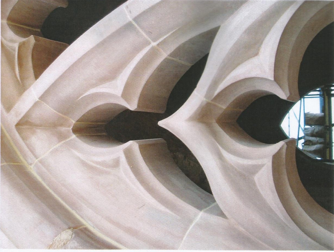
4. Renewed tracery to belfry light
