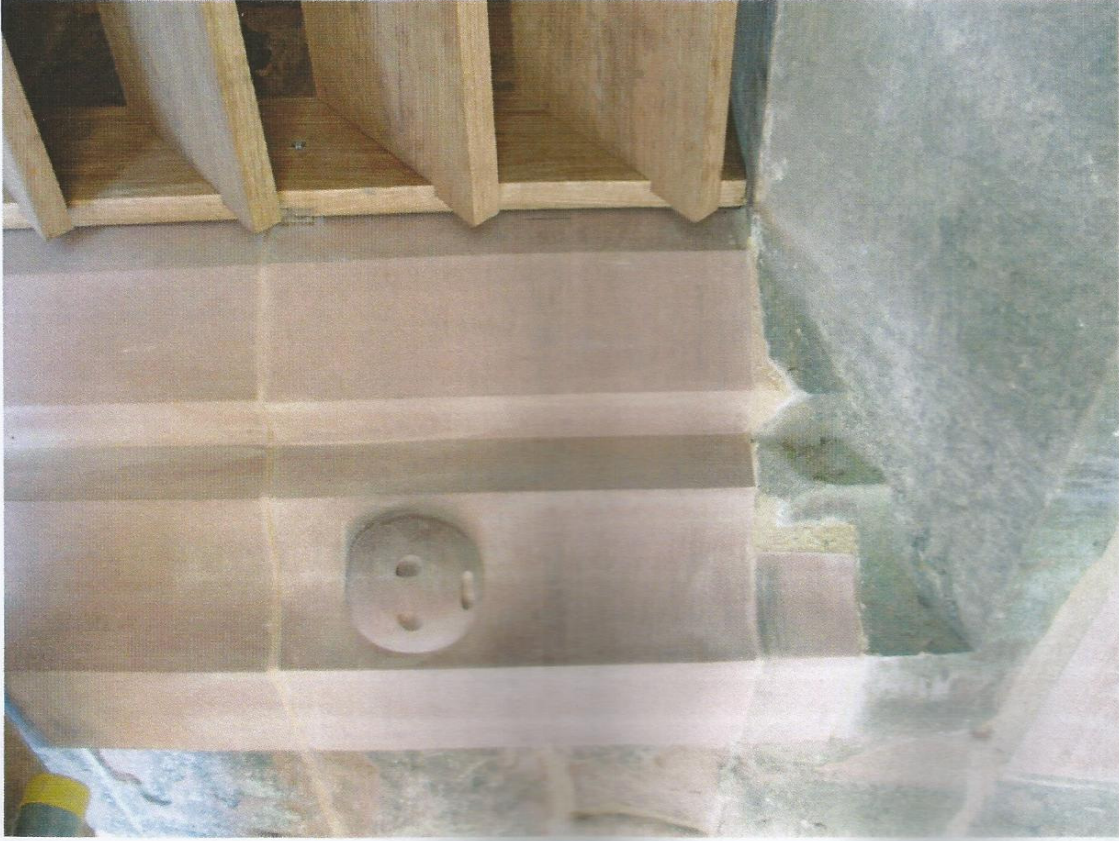
1. Renewed stonework to jamb of spire light and new oak louvres
