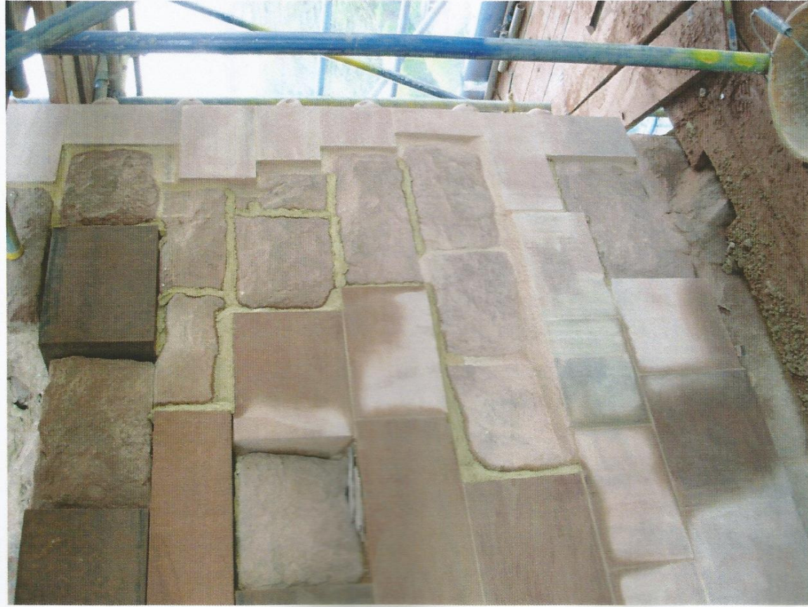
5. Re-building of quoin at belfry stage
